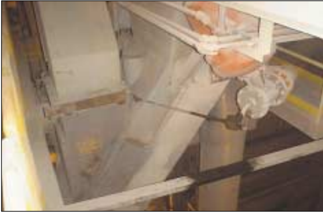
Raw feed inlet chute.
